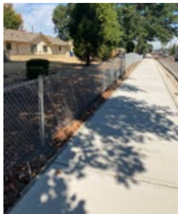
Example of recent sidewalk project M St SE, completed in early 2022
